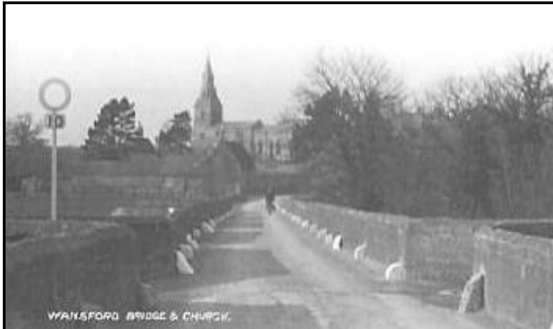
Note the 10 mph speed restriction! As the projecting hubs of cart wheels would score bridge parapets, stones were set to protect the walls so that the wooden wheels of passing carts risked significant damage if driven too close
